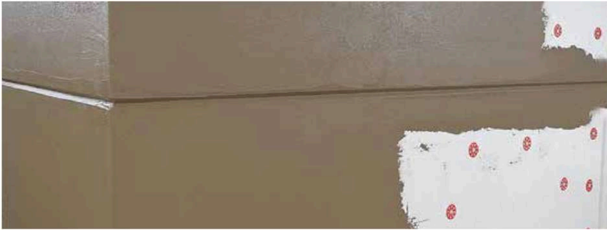
First coat of Raso Top 800 basecoat
