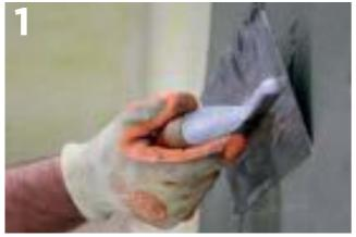
With the help of a notched trowel (4 mm) spread special Basecoat adhesive on a substrate of approximately 1m2. Do not spread on wider area due to fast drying rate of the adhesive. Thickness of the layer should be around 2 mm. It is recommended to start where the first tile is to be installed and working across horizontally to complete at least one full row of brick slips.
