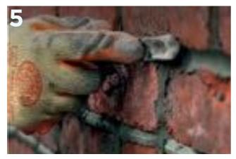
After pressing the brick slips the fresh excess adhesive must be removed by using a brush (12 mm wide) .It is very important to pay attention to the execution of sealing the joints to block the access of the water between the brick slips and the adhesive. It is very important to cover the edges of the brick slips must be fully coated with the adhesive.
