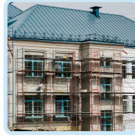
External Wall Insulation
