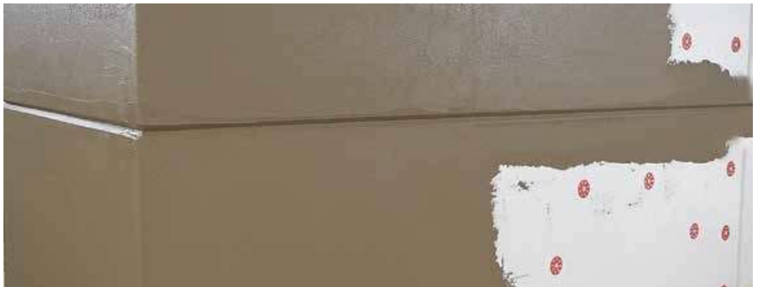
First coat of Raso Top 800 smoothing compound
